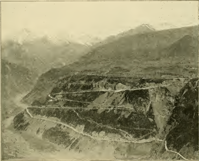
How the Georgian Road Comes Down at Mleti.
